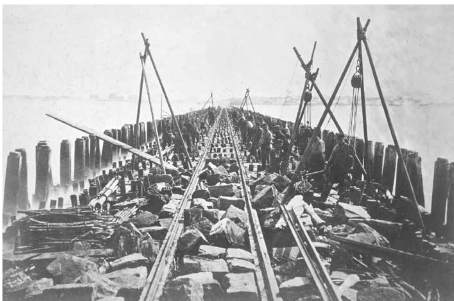
Construction of the Northern Mole at Hoek van Holland, situation in 1871
