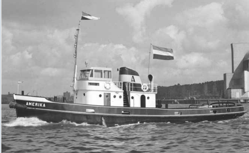
A post-WW2 first-generation 610 bhp shiphandling tug built 1952 for P. Smit Jr photo: coll. Job van Eijk
